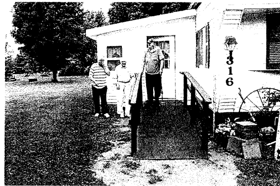
Jack Hensley standing on his newly constructed ramp to allow easier access to his house.
